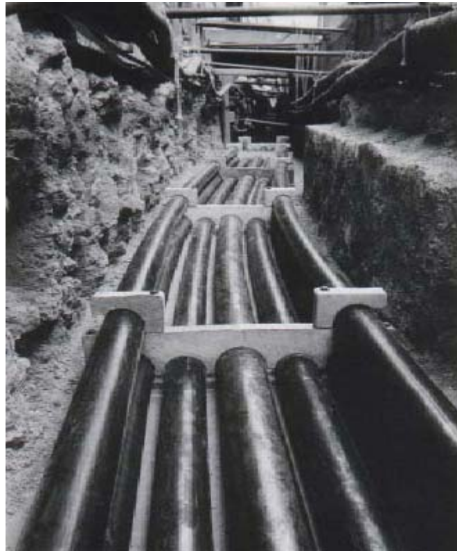
Figure 69 Laterally cooled UGC in Vienna with four cooling pipes (two between cables and two above outer cables)
