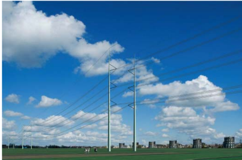
Figure 6-13 Wintrack tower design for reduced magnetic field levels under 400 kV lines (source TenneT)
