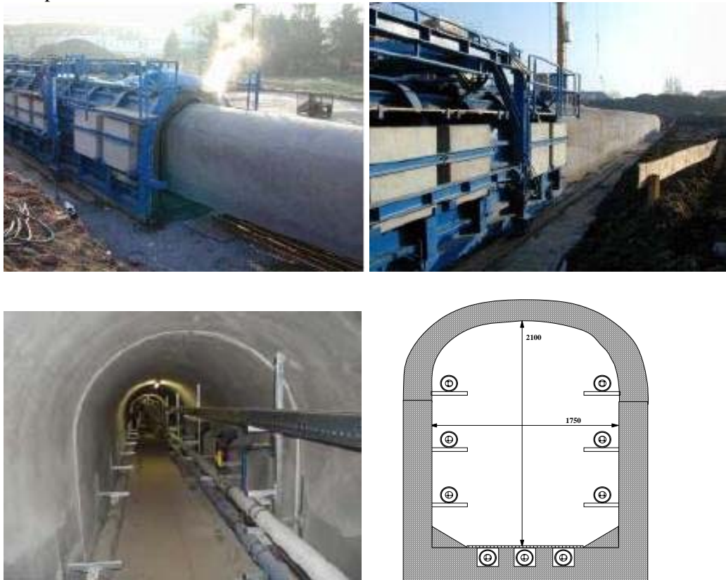
Figure 75 Infrastructure tunnel, system Dupré, Speyer; above: construction works, below left: installation of equipment in the tunnel, below right: schematic drawing of tunnel cross section with three UGC circuits
