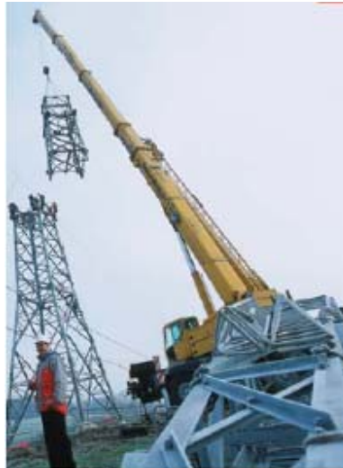
Figure 4-2 Assembling of preassembled steel segments by the use of a mobile crane (source: E.ON Netz website)
